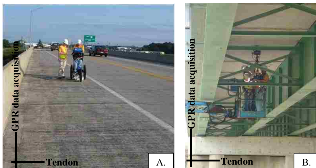
Figure 3.7: Process of acquiring GPR data in the longitudinal direction (A. Top surface acquisition using a cart, B. Bottom surface acquisition using a survey wheel apparatus)
